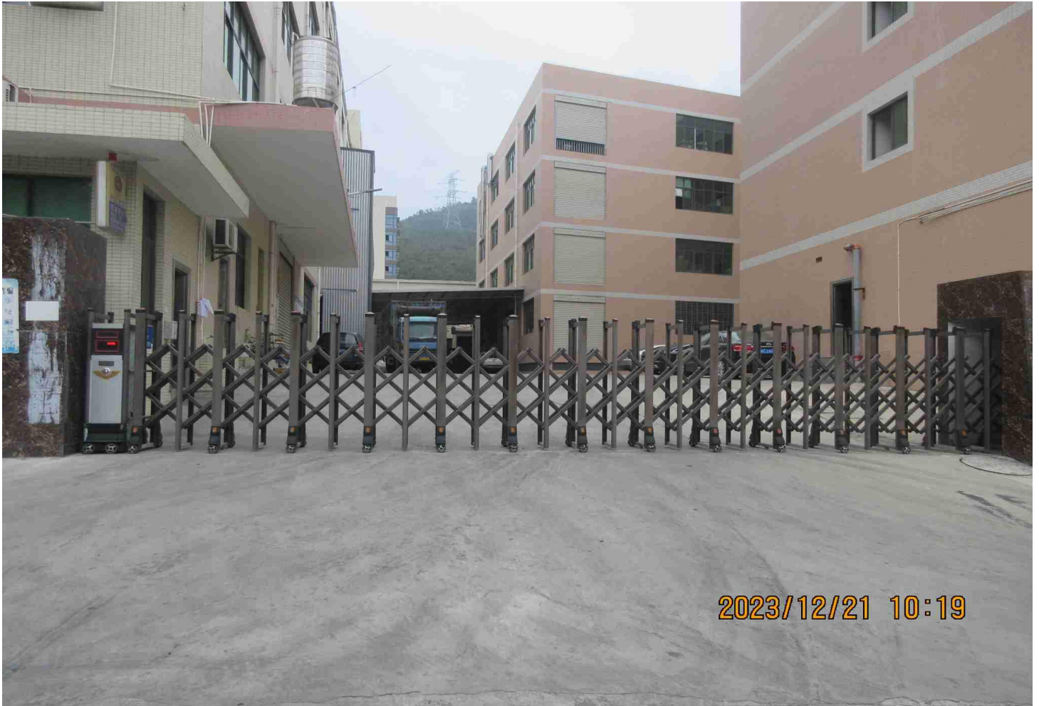
Barriers to control ingress and egress.jpg
